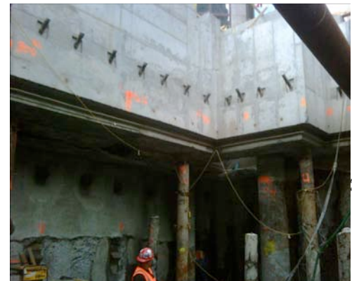
Excavation and foundations for tunnel
